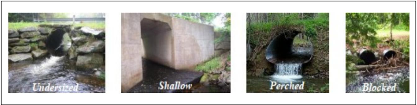
Barriers to fish passage include undersized, shallow, perched, and blocked culverts and bridge openings
